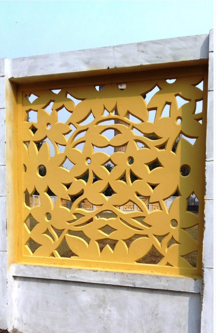
GRC jaali at BHEL park,GHZ.
